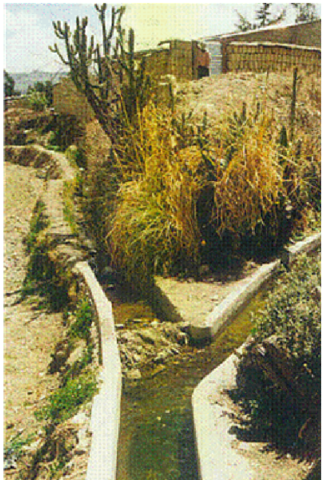
Strong irrigation channel in the Achocalla Community Photo: H. Timmer
